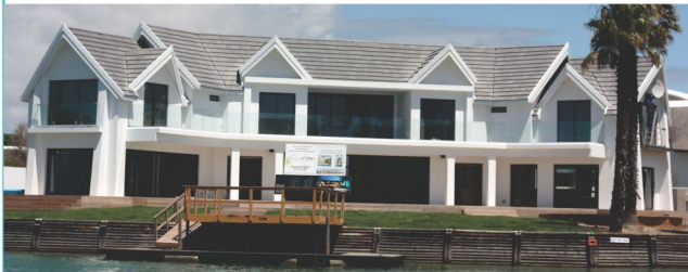
One of the stunning, mansions being built on the St Francis Bay canals - after the 2012 fire... This one, almost complete, is being built by Willem du Bruin. See story p2
