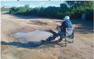
Cape St Francis residents are angry about the crater-size potholes in Da Gama Road. One resident decided to see if he could find some fish in one of the ponds after the rain. Photo: Avery Whitehead.
